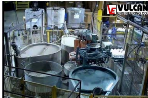
Robotic Cluster Coating Unit
